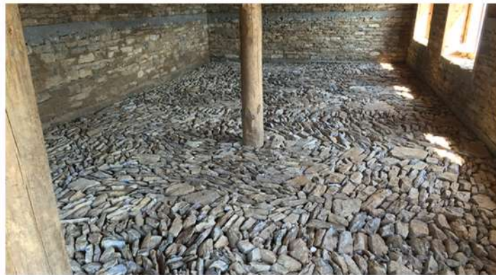
▲ Panoramic view of the construction site.
