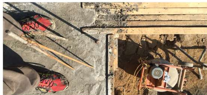
Building under construction. ▶
